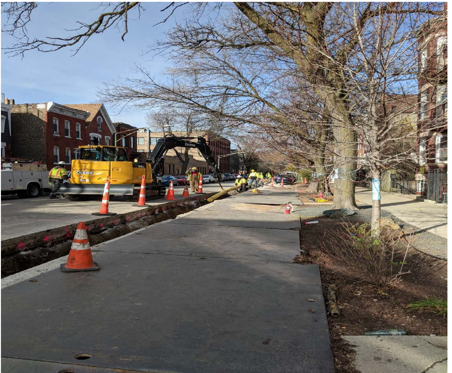
Milwaukee Phase 1 - Open Cutting 8" Medium Pressure Main at 1600 N. Honore
